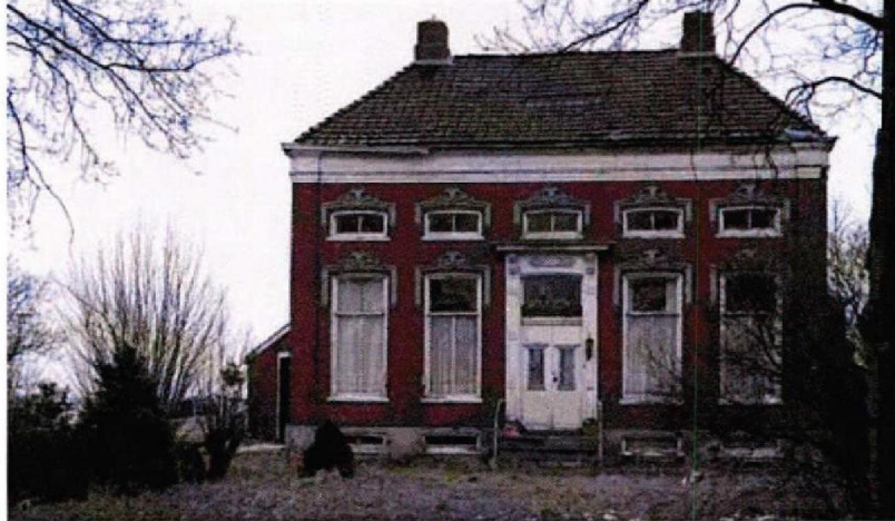
Figure 4.7 Example of a dilapidated building. Illustration taken from "VROM-Inspectie, Handreiking aanpak vervallen panden", April 2007 (Ref. 18).
