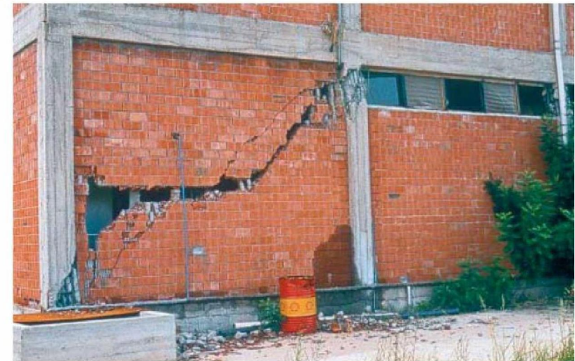
10/1 This structural stairway wall will be destroyed by a relatively weak earthquake. A total collapse of the building may result (Switzerland 2001).
