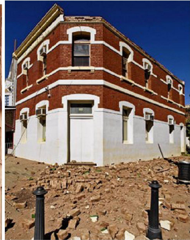
Parapet (Borstwering) Kalgoorlie, Australia 2010 Magnitude 5 Depth 2km
