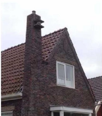
Figure 18 Example of a chimney with ornament.
