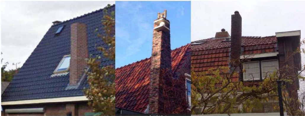
Figure 16 Examples of slender chimneys.
