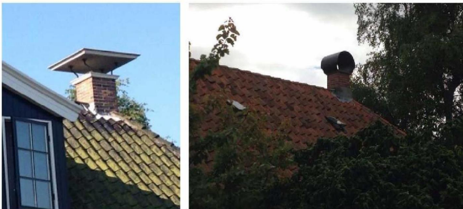
Figure 17 Example of chimneys with caps.
