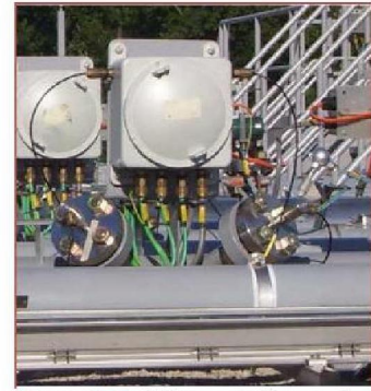
Figure 4.6 – Ultrasonic flow meter
