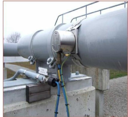
Figure 4.2 – Sand detector mounted on a flowline
