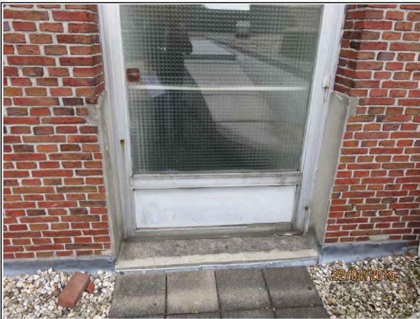
Schade 17, Verticale scheuren (57784 22-4 (184))
